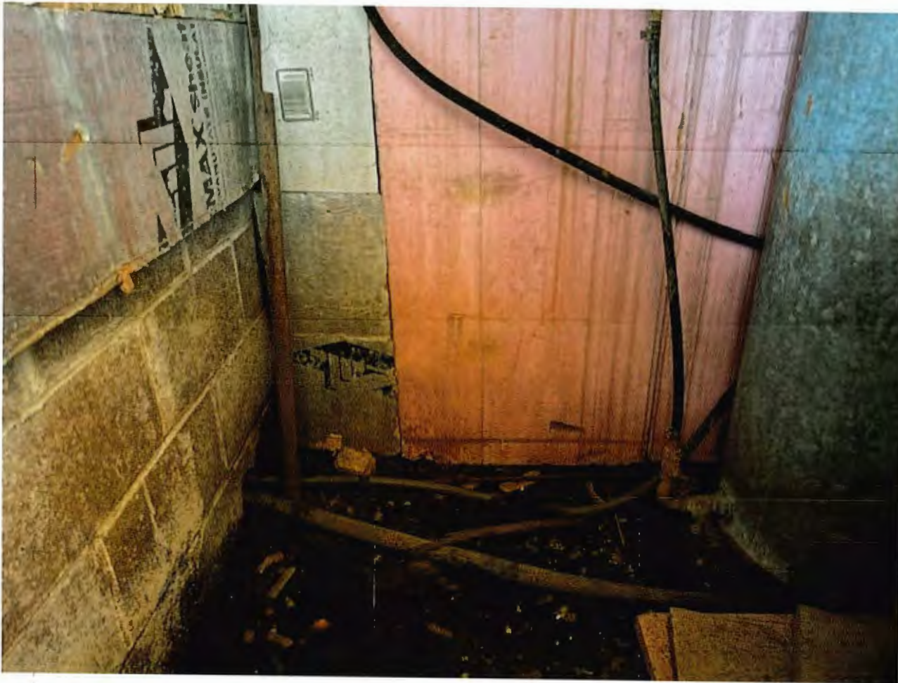
Existing foundation Below stairs
