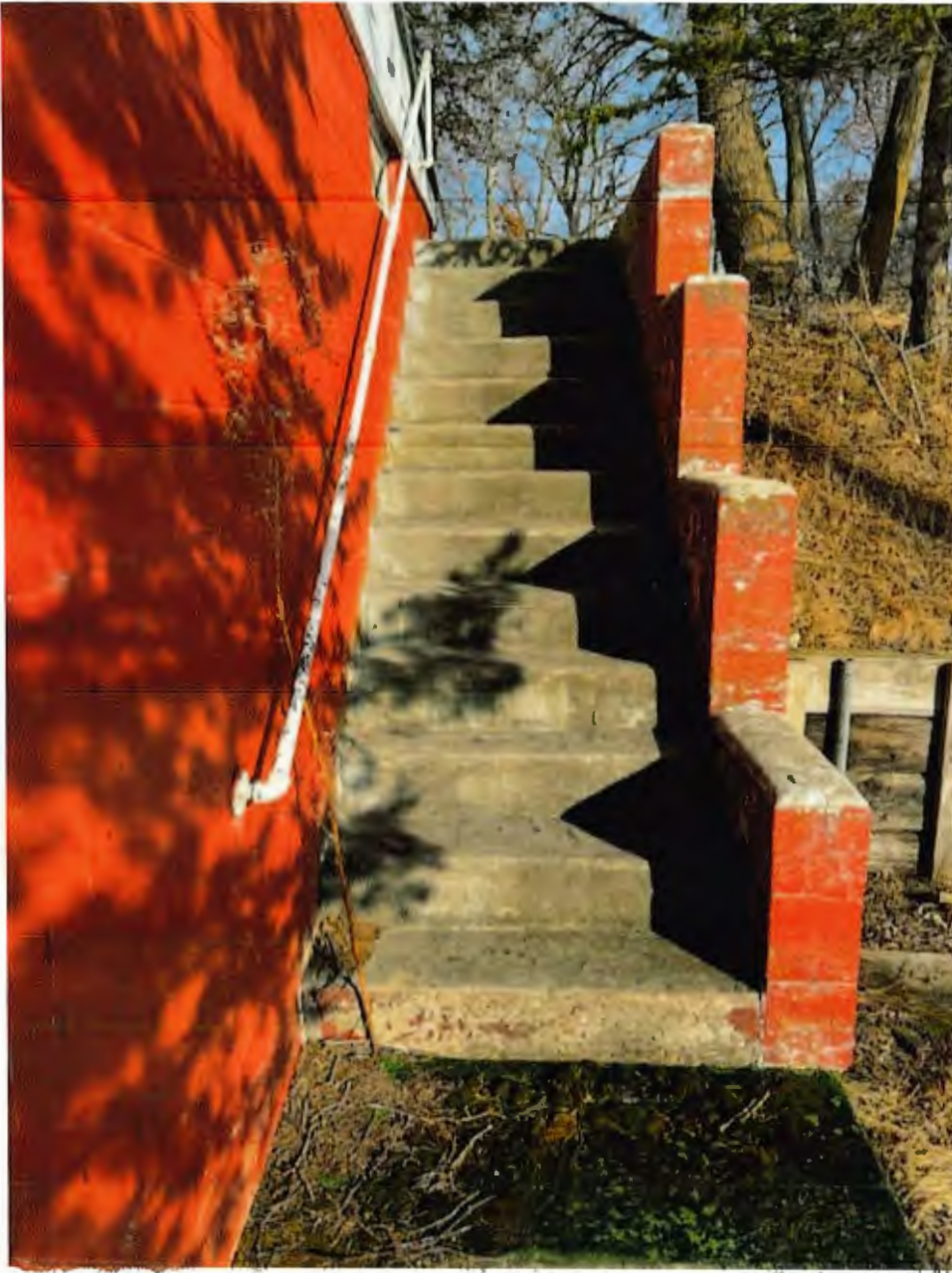
Existing Stairs "Impervious Surface"
